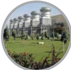
Parand Combine Cycle Power Plant
