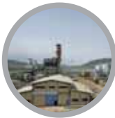
Khoi Power Plant
