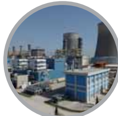
Kazeroun Power Plant
