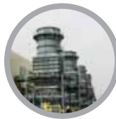
Ardebil Gas Power Plant
